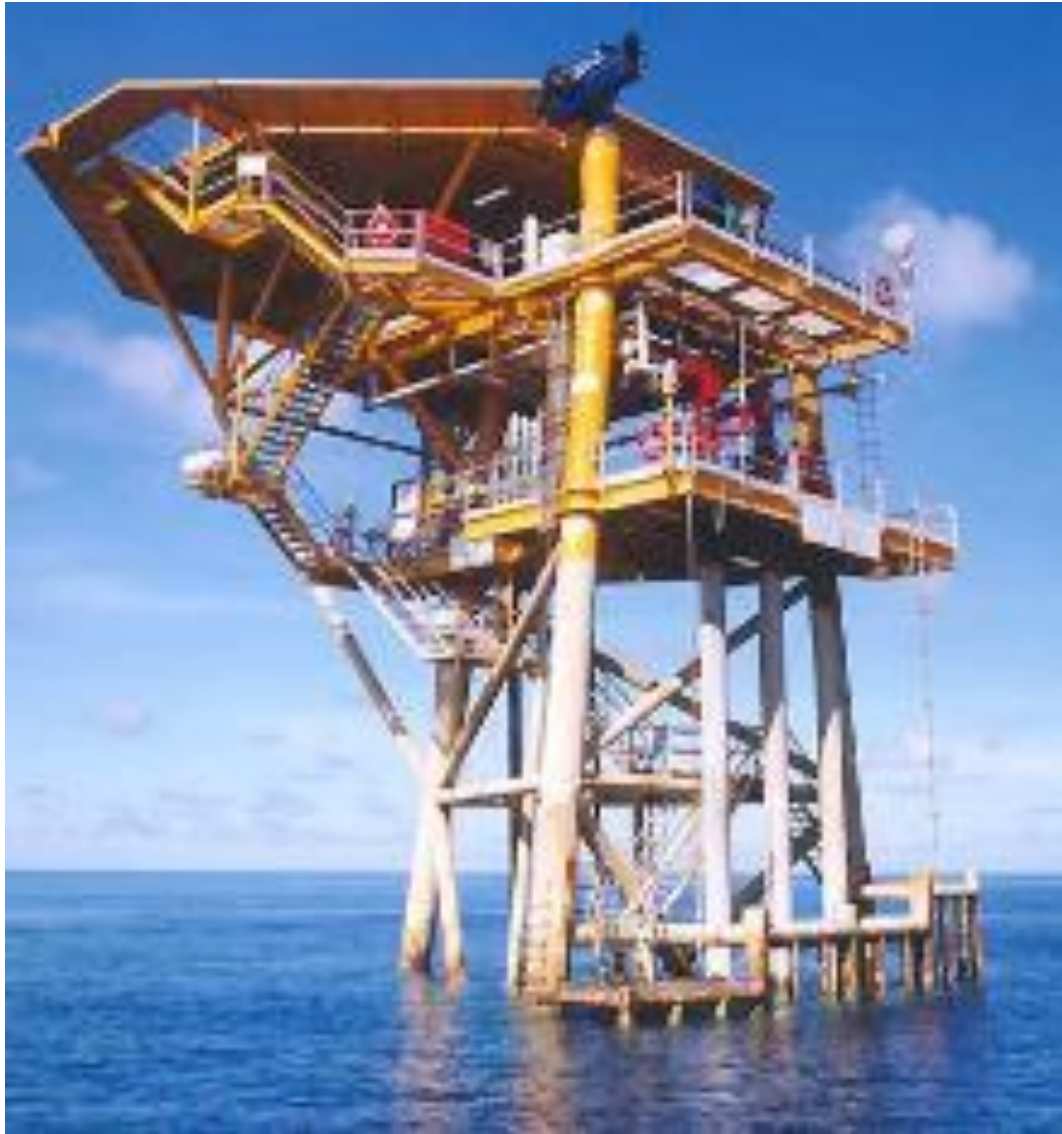
Figure A-2 Not Permanently Attended (NPAI) helideck
