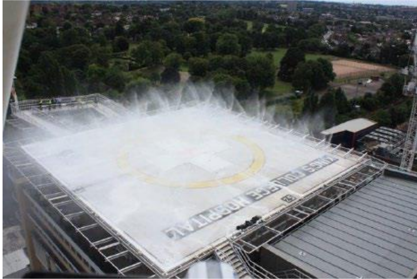
Figure 16-3: A foam DIFFS on a solid plate deck surface
