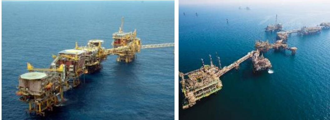
Figure A-1 Fixed platforms with helidecks above accommodation
